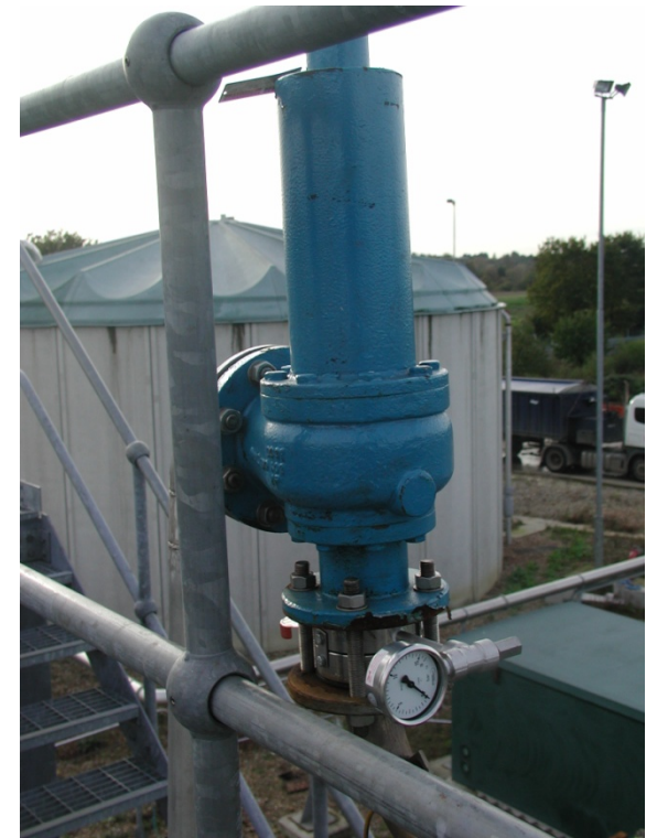
Pressure relief valve with bursting discs
