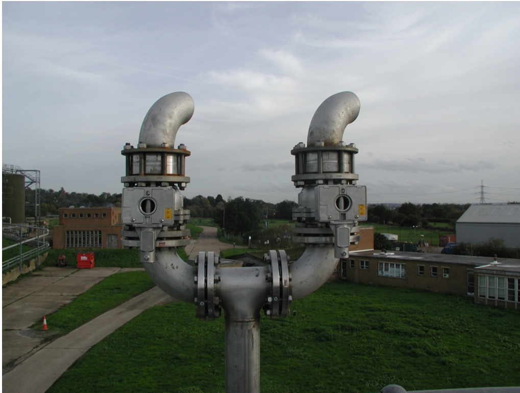
Vacuum break valves with bursting discs, in locked position
